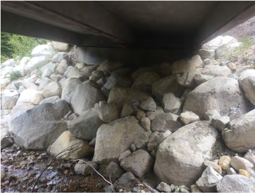
Right Bank Abutment when facing downstream
