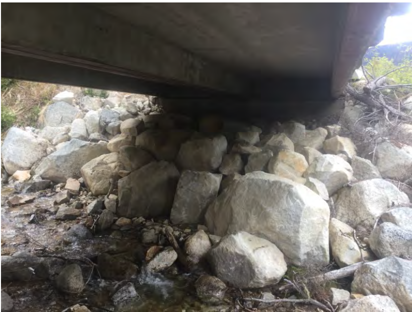
Left Bank Abutment when facing downstream
